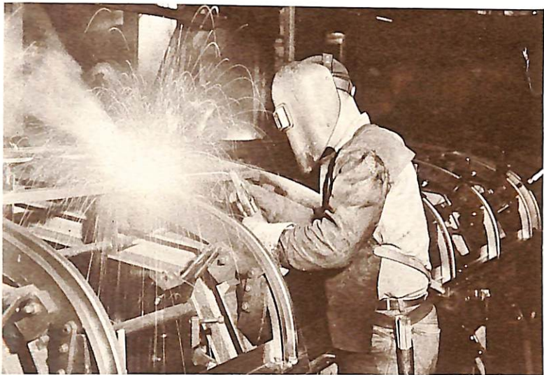
Steel welds steel for utmost strength as the roof frame members locked in this precision jig are all welded into one complete unit. Sturdy, one-piece roof bows assure maximum strength in event of a roll-over.
