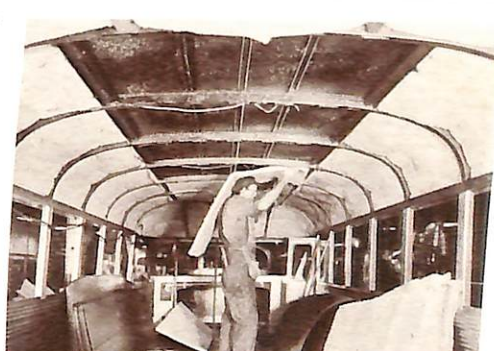
Thick spun-glass insulation for extreme climates gives added protection against heat and cold. Optional extra.
