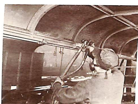
Double, sprayed-on roof insulation. Covers both outer and inner panels as buffer against heat and cold.
